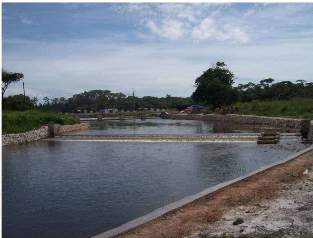
Rehabilitated spillway at NARDC
