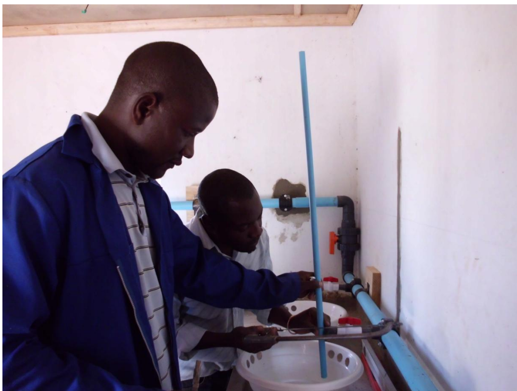
Mr. Chad Kanchea and Mr. Given Kujila constructing a Tilapia incubating facility at Fiyongoli Aquaculture Research Station, Mansa.
