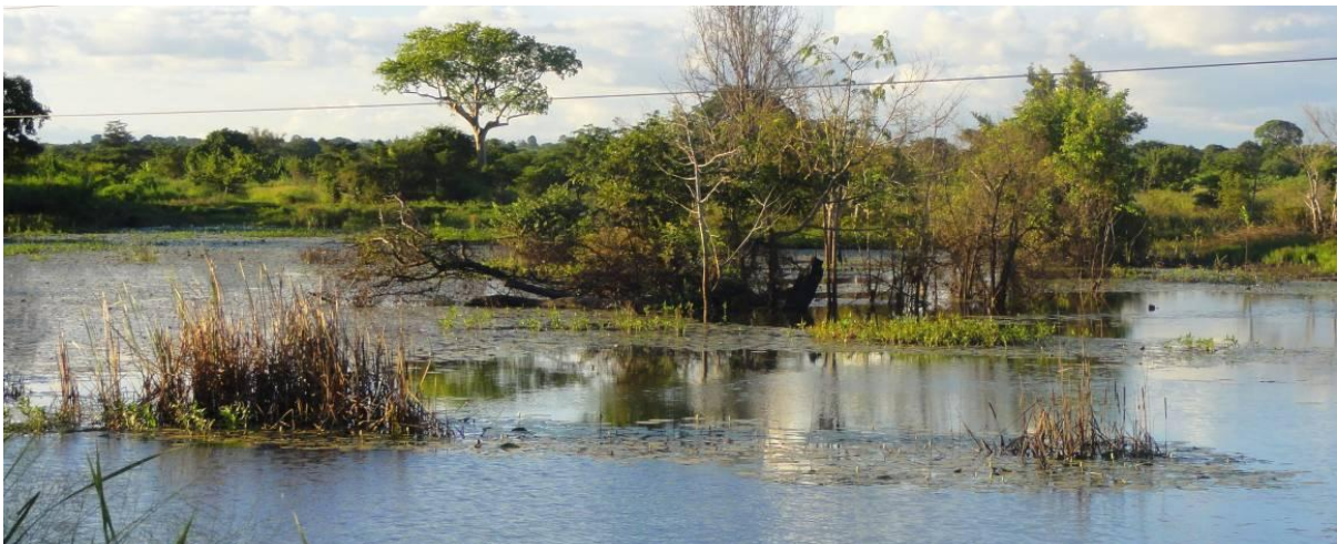
Figure 5.4: Small pond on Malipe Stream caused by road embankment on road to Balama.
