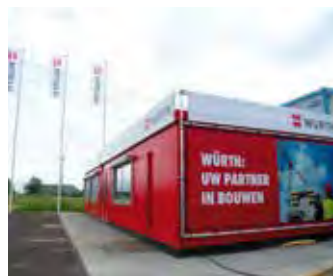
Service-shop Stationair magazijn
