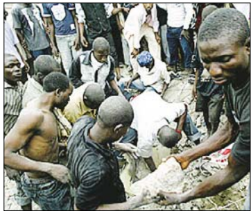
Rescue workers search through the rubble of a collapsed building in Lagos.
