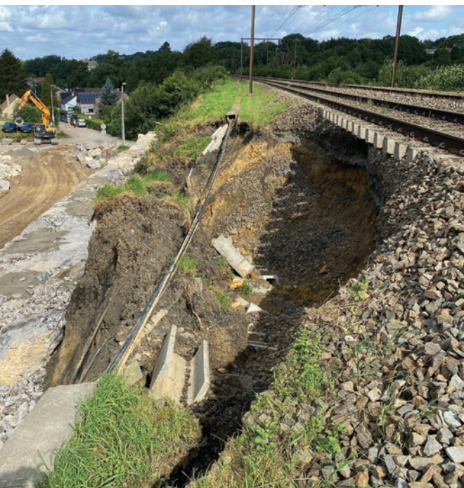
Innovative methods were needed to repair the embankment collapse at Mont-St-Guibert.
