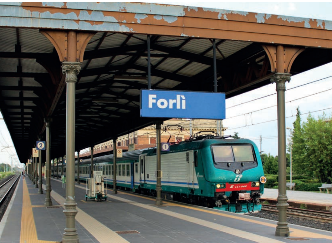
Among RFI's investment programmes is a modernisation of the Adriatic Corridor down the eastern side of the country.
