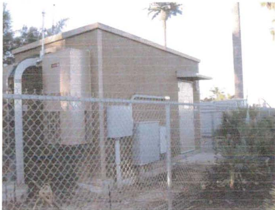
9. Shelter from northeast
