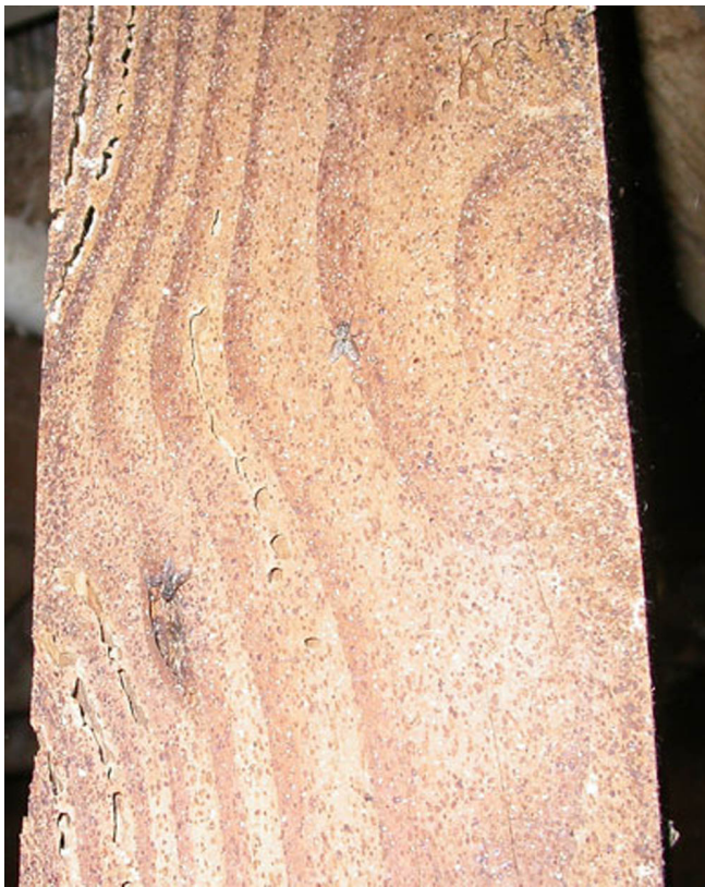
Figure 10. Damage on wooden pillar caused by larvae of the lesser mealworm, Alphitobius diaperinus (Panzer). Credits: Cornell University
