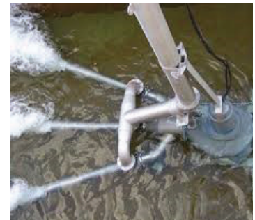
Jet aerator in the water with an efficiency of: SAE: 2.4 kg O 2 /kWh
