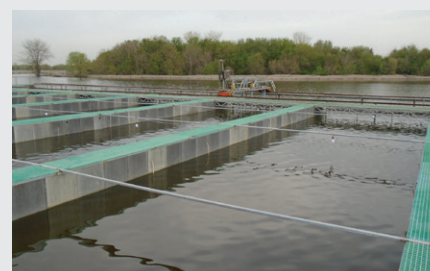
FIGURE 3-9: RACEWAYS OF AN IN-POND RAS
