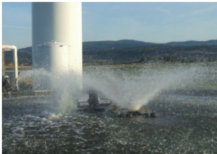
Spray aerator with an efficiency of: SAE: 0.06-0.17 kg O 2 /kWh
