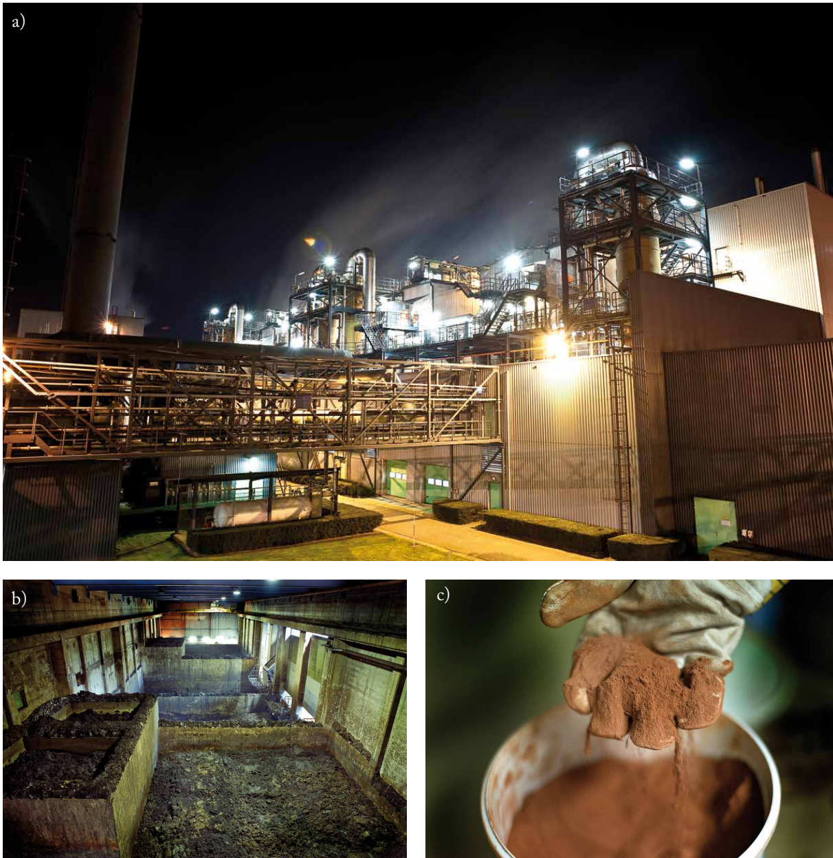
Figure 7.2 a) N.V. Sluiverwerking Noord-Brabant (SNB) in Moerdijk; Europe's biggest mono-incineration plant. Here, biosolids from wastewater purification in the water treatment facilities of both regional water boards and commercial parties are incinerated. b) Storage of ~16,000 tones of phosphorus-rich biosolids awaiting incineration and further processing. c) Phosphorus-rich ashes from the incineration of biosolids which can be used to make recycled fertilisers. Photographs taken by Nils Laenger - http://nilslaenger.de/
