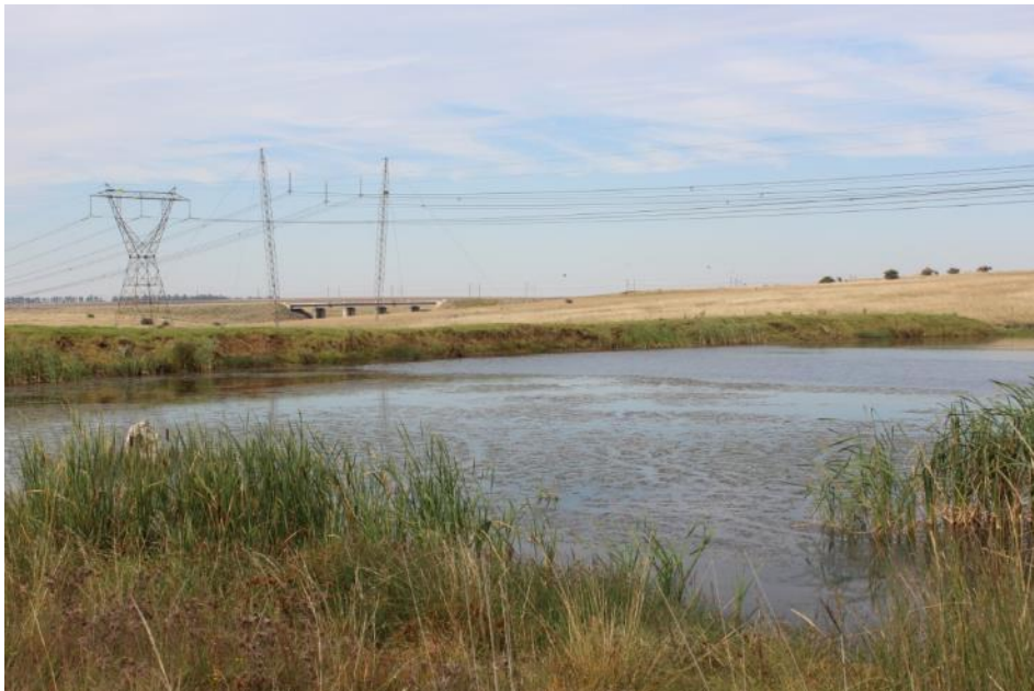
Figure 35: A manmade dam on the study site. Note the N17 Bridge in the background.
