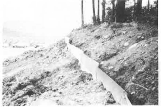
Figure 8. Upper drain partially backfilled.
