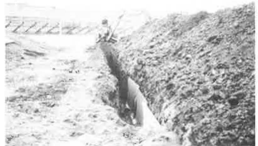
Figure 10. Installing lower drain in trench.
