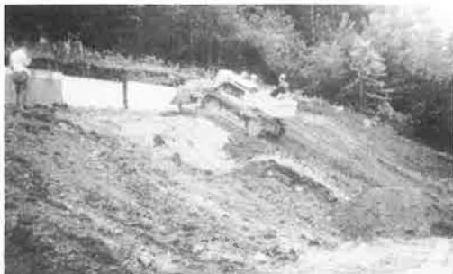
Figure 9. Dozer backfilling upper drain.
