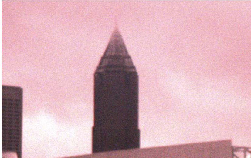
Figure 348. Nov. 30, 2010 Visible Image of Bank of America Building taken with the Hyper-Cam.
