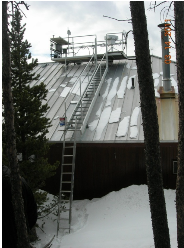
Figure 171. Rooftop platform on base camp building and access ladder/stairs.
