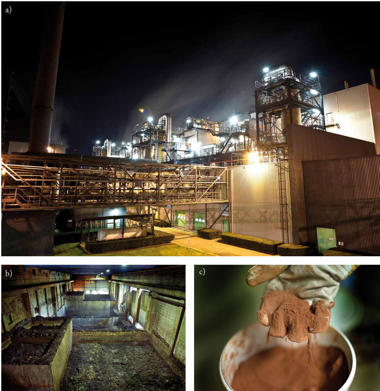
Figure 7.2 a) N.V. Slibverwerking Noord-Brabant (SNB) in Moerdijk; Europe's biggest mono-incineration plant. Here, biosolids from wastewater purification in the water treatment facilities of both regional water boards and commercial parties are incinerated. b) Storage of ~16,000 tones of phosphorus-rich biosolids awaiting incineration and further processing. c) Phosphorus-rich ashes from the incineration of biosolids which can be used to make recycled fertilisers. Photographs taken by Nils Laenger - http://nilslaenger.de/
