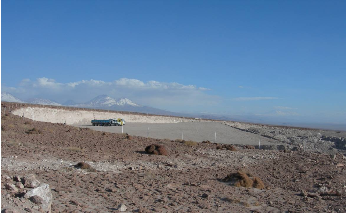
Earthworks completed at OSF.
