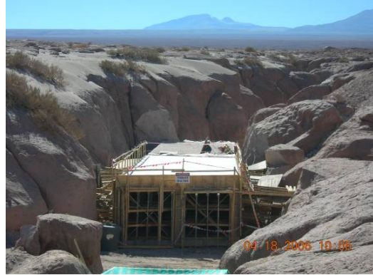
Concrete works complete.
