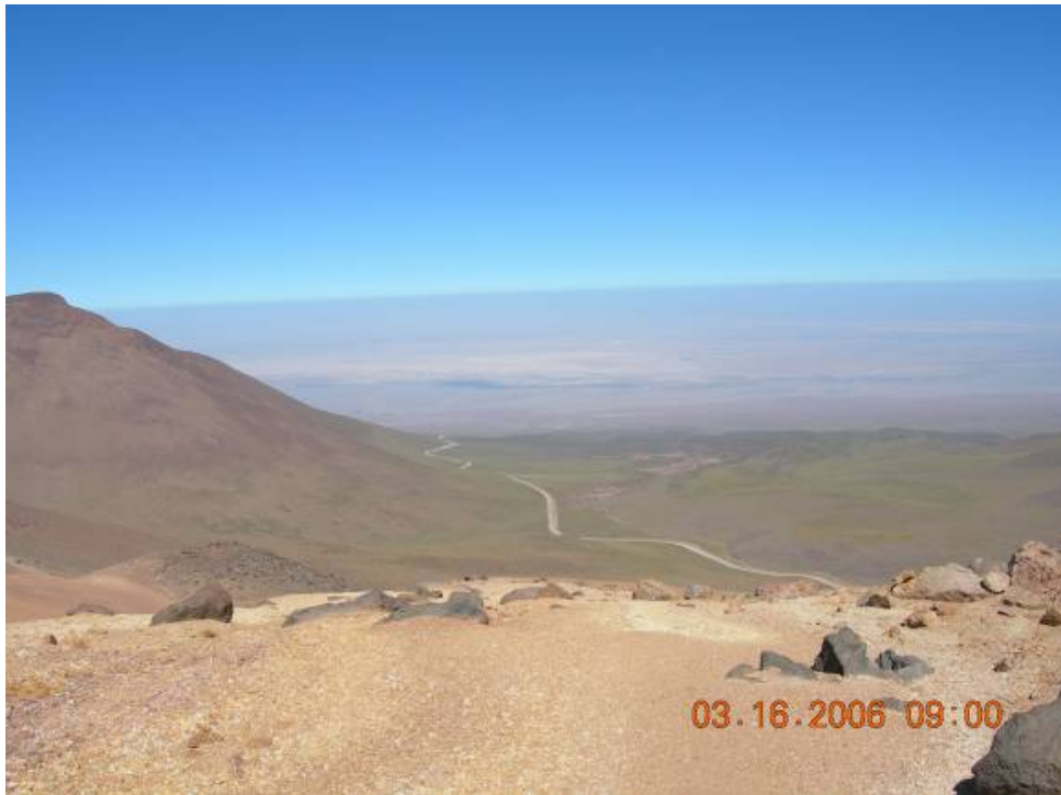
Road completed to final width.
