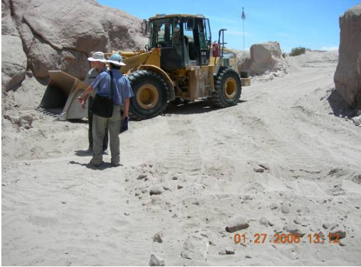
Construction of culvert.
