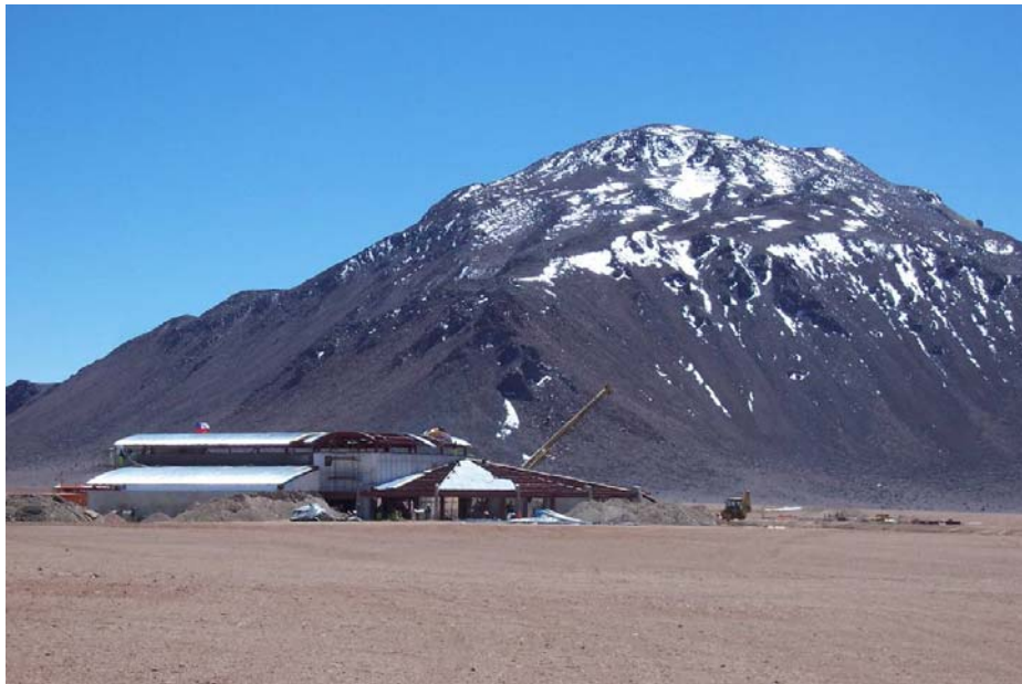
AOS Technical Building.
