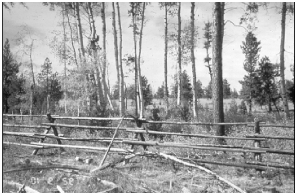
Figure 1 —Buck-and-pole livestock exclosure made from native lodgepole pine. Note the successful aspen regeneration inside the exclosure.
