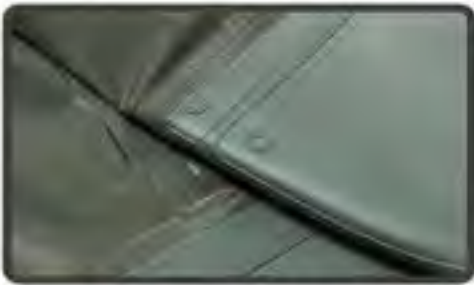
Heat Welded Seam
